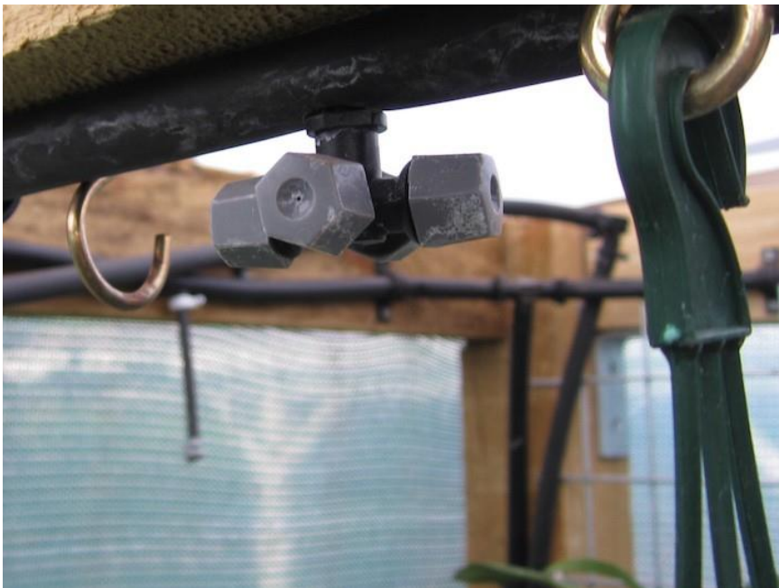
Figure 4. The automated watering system comprises a combination of overhead misters (foreground) and under bench sprays for cooling and raising the humidity and micro sprays (background) for watering.
