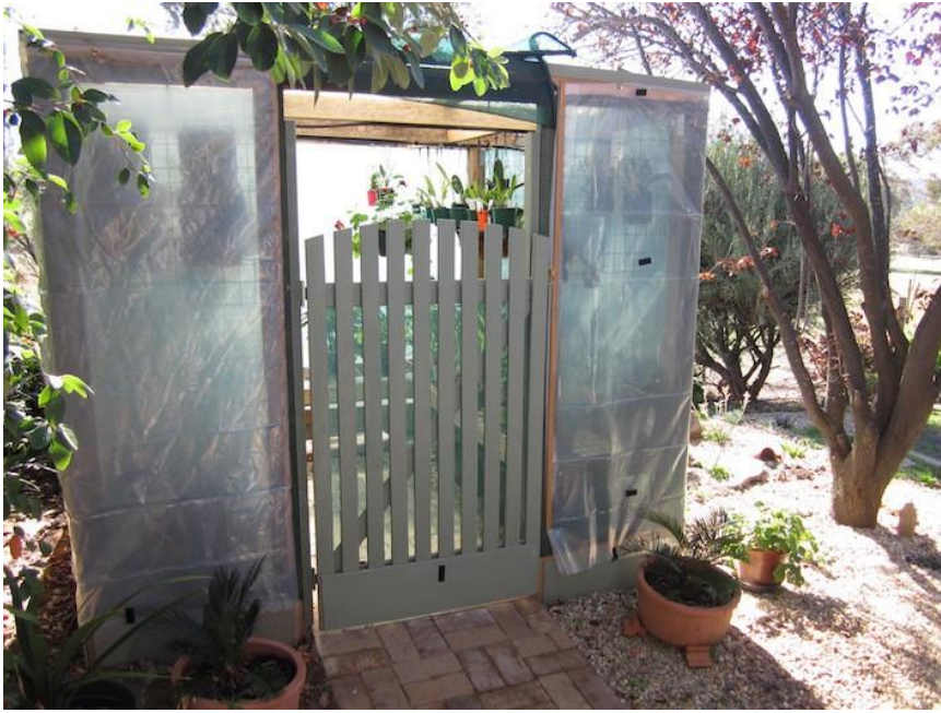
Figure 1. Shade-house consisting of treated pine frame with polycarbonate roof and shade cloth slides. The shade-house is wrapped in removable horticultural film secured with Velcro in cooler months with a door flap that can be folded back to prevent overheating. The deciduous tree on the eastern side shades in summer but allows the sun in during autumn-winter.
