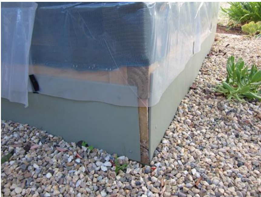
Figure 2. Base of shade-house is closed in with fc fibre-board to increase humidity.
