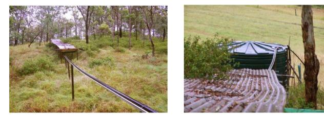
This device is almost as good as a bore during a wet period as it collects every drop of rain or dew that falls on it and feeds it into the tank, greatly supplementing the dwindling supply from the bore. Other
