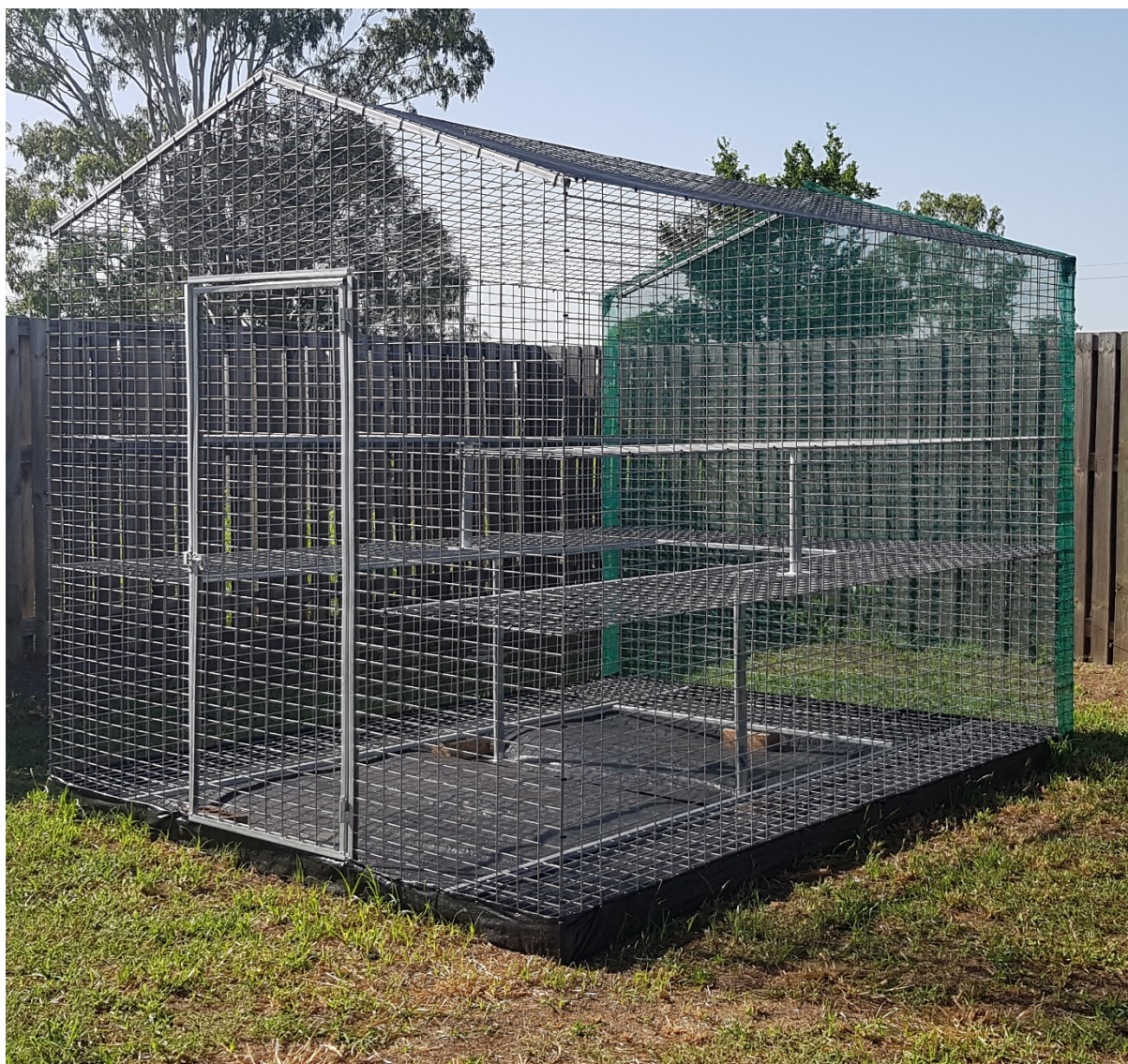
My 2.5 m wide x 3 m long shadehouse in the process of attaching shadecloth.
